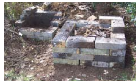
The Block Bin System: Rebuilding the Bin.
