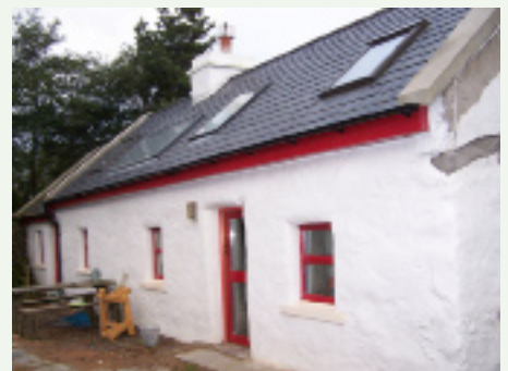
Cottage rebuilt for under €40,000
