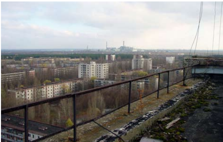
The abandoned city of Prypiat (population formerly 50,000) with Chernobyl in the background
